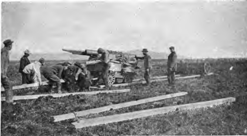
GETTING A SMALL PUMPING PLANT OVER THE TUNDRA TO A FRESH WATER LAKE, TO PUMP WATER FOR OUR LARGE ENGINES.
